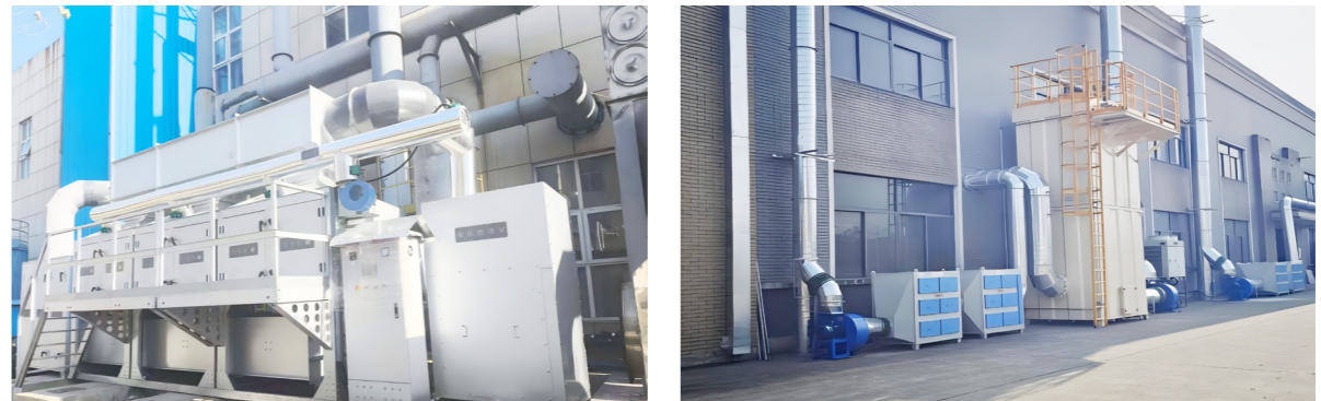
Environmental Protection Equipment Upgrade and Retrofitting
