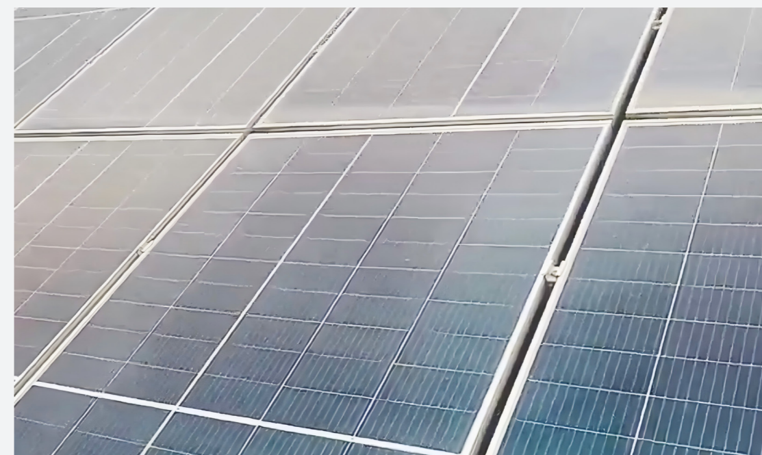
Anhui Boster installs photovoltaic panels
